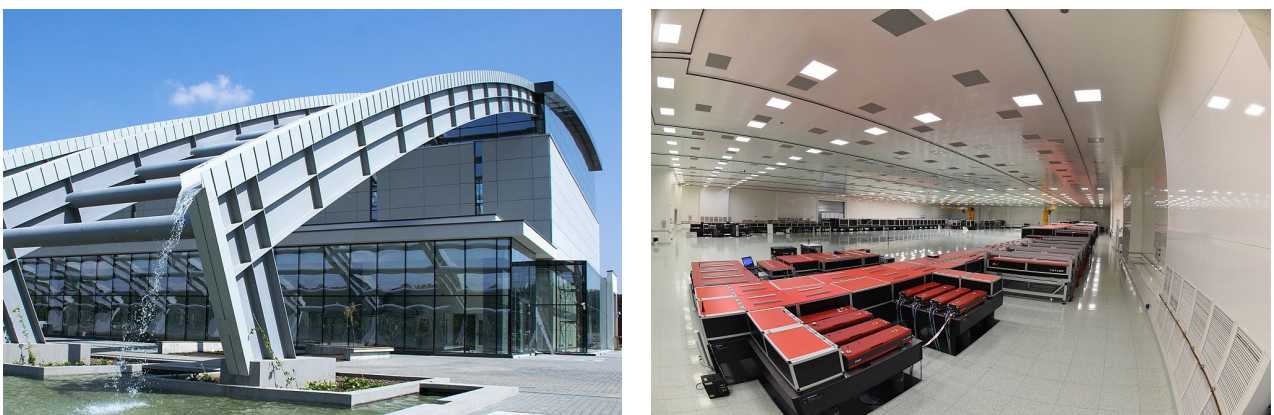
Figure 34: Extreme Light Infrastructure – Nuclear Physics at Magurele, Romania. Left: Part of the Experiment Building housing the two 10 PW lasers and the VEGA system; Right: the laser hall of the 10 PW lasers.
